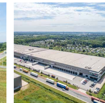
SMARTLOG AMSTERDAM CONAKRYWEG 1 CONSTRUCTION YEAR 2019 43,000 M 2
